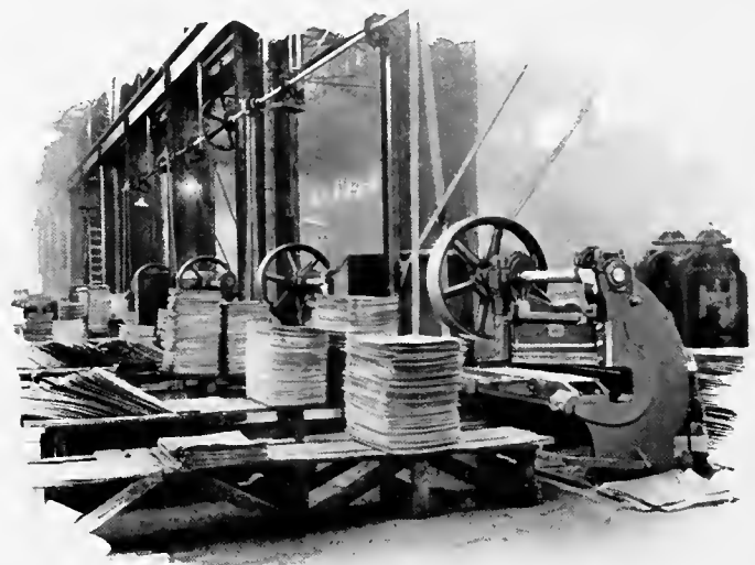
Installation of Mesta Squaring Shears in a Tin Mill
